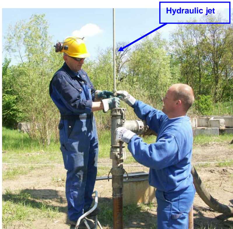
Figure 4. Notch the borehole by applying a trio of hydraulic jets.
