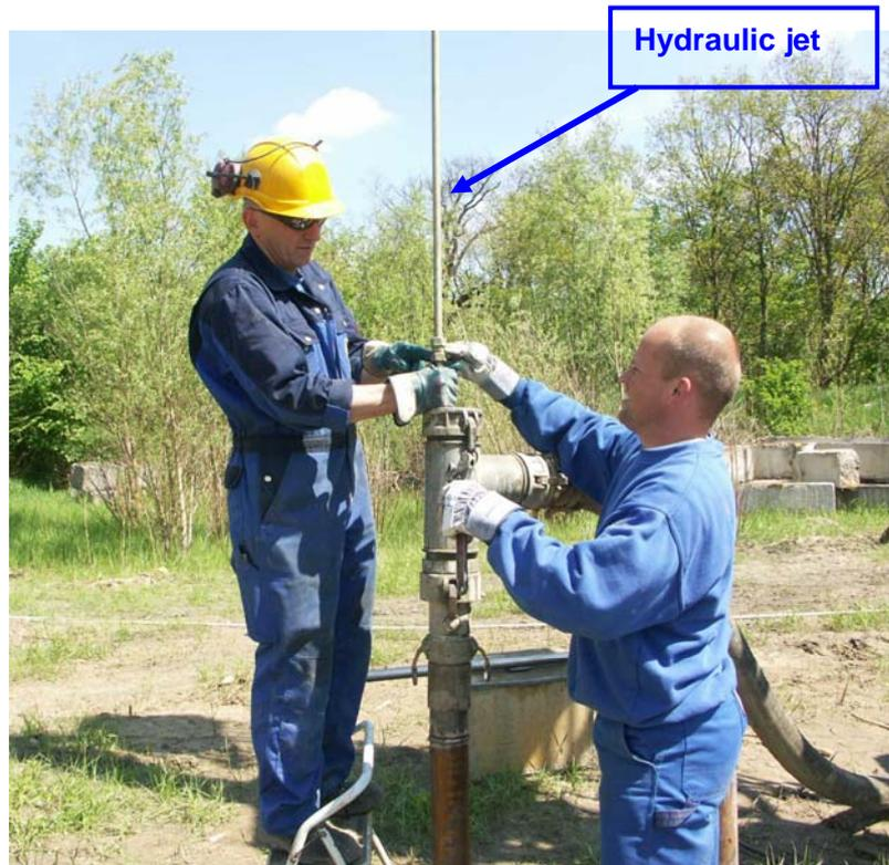
Figure 4. Notch the borehole by applying a trio of hydraulic jets.
